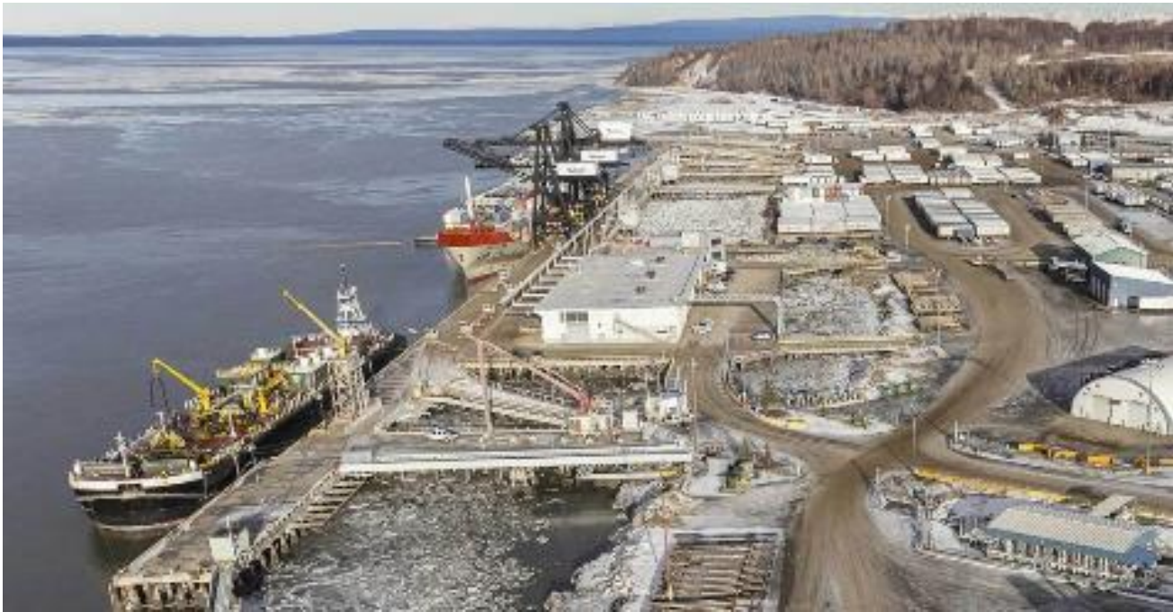
Figure 33: Port of Alaska (Anchorage). Image Source: Northstarak.com
