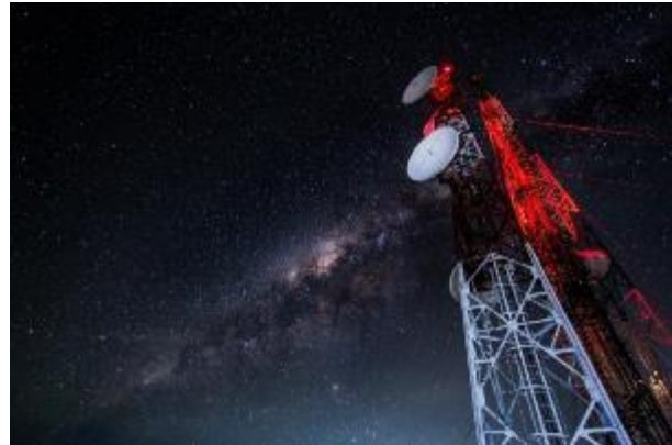
Figure 60: Communications tower. Image Source: Pixabay
